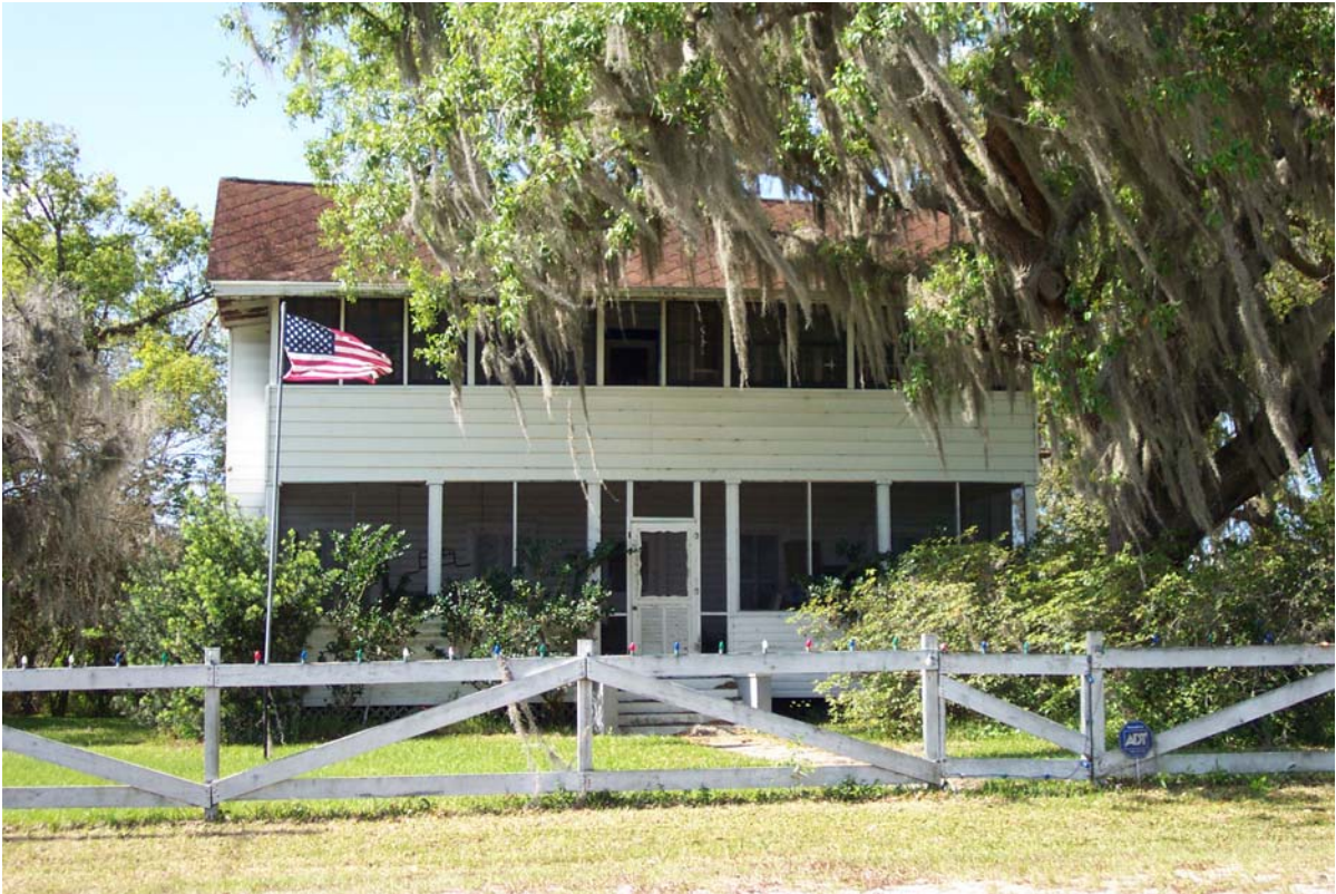
Figure 5.25 MA01609-Youngblood, R. Page-12251 CR 675 (Rutland Rd.) - Current Photograph Renker Eich Parks Architects
