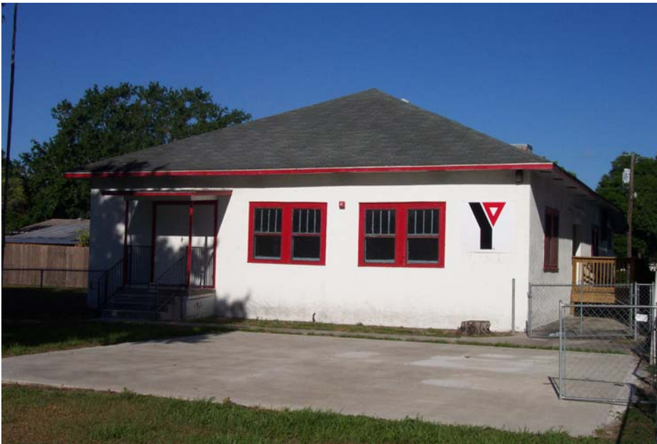
Figure 5.23 MA01593-YMCA-7006 122nd Ave. E. – Current Photograph Renker Eich Parks Architects
