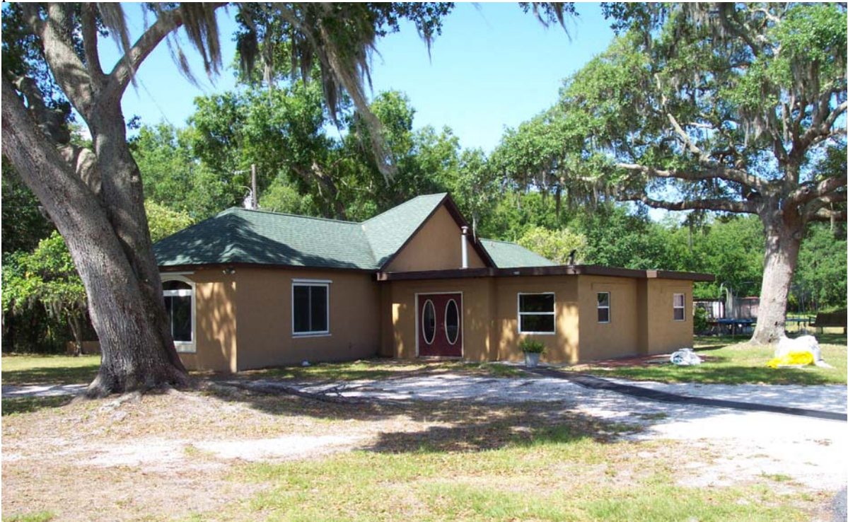
Figure 5.26 MA01617-Lemieux, John - 5015 Fort Hamer Rd. - Current Photograph Renker Eich Parks Architects
