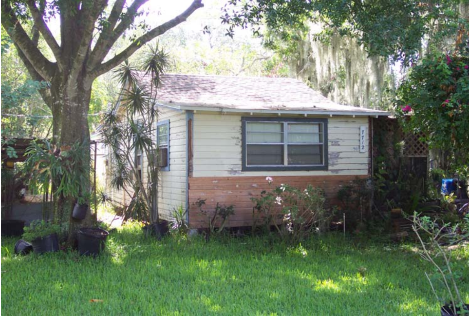
Figure 5.22 MA01588-Williams, Maxene B. - 7712 122nd Ave. E. – Current Photograph Renker Eich Parks Architects
