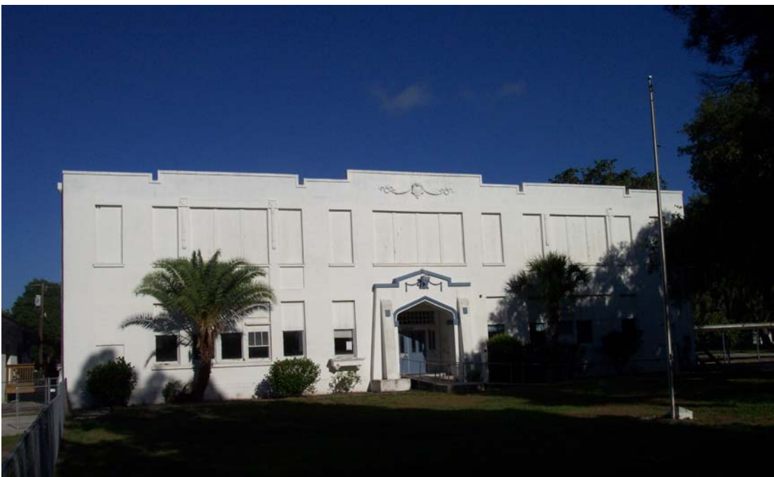
Figure 5.6 MA00764-Parrish School-12214 US Hwy 301 N. - Current Photograph Renker Eich Parks Architects
