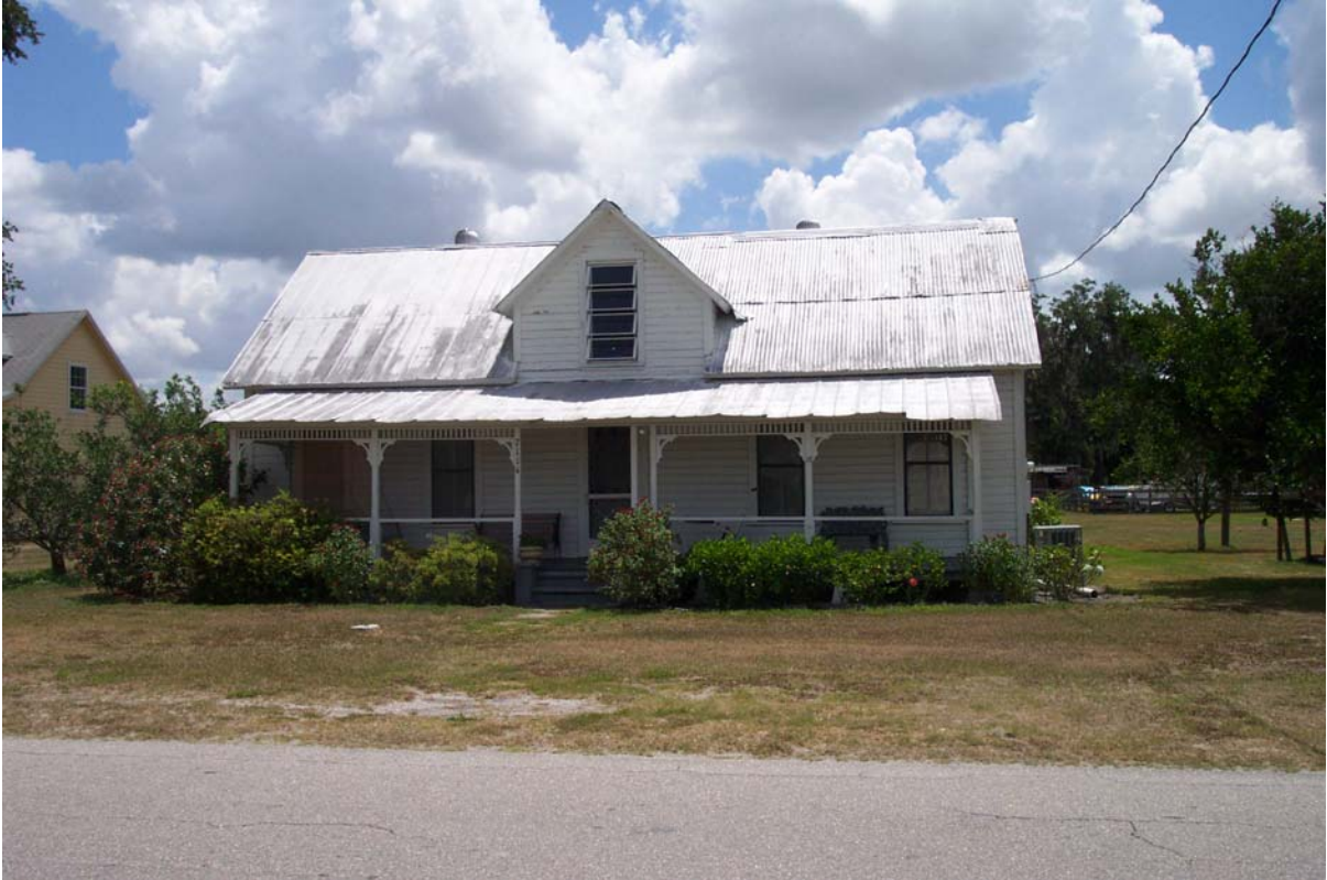
Figure 5.20 MA01563-Buice, Clarence M.-7114 121st Ave. E. - Current Photograph Renker Eich Parks Architects
