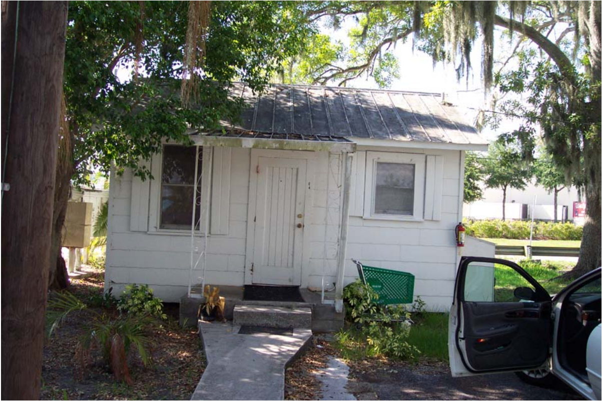
Figure 5.28 MA01629-Waterfront Ventures - Cabin 4-6015 18th St. E. - Current Photograph Renker Eich Parks Architects
