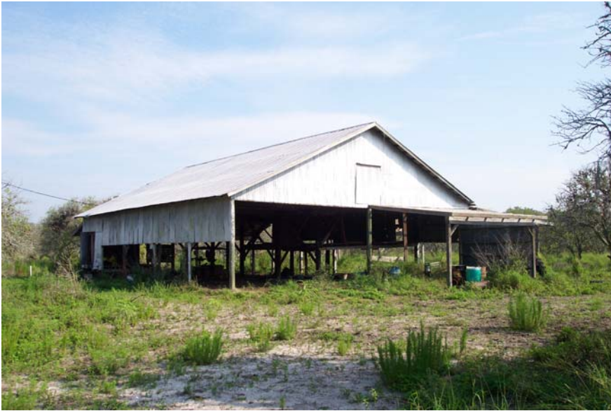
Figure 5.12 MA01348-Cone Barn-12323 State Rd. 62 - Current Photograph Renker Eich Parks Architects
